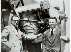
George & William Besler pose with their installation showing the compact boiler system. It was calculated that just 10 gallons of water would be sufficient for a flight of 400 miles. According to these two experimenters bv increasing the size and efficiency of the condenser, they believe they can make this amount of water last indefinitely ?? (Sketch below
