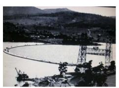
The gantry was placed at one end to allow the passage of shipping passing up and down the river.
