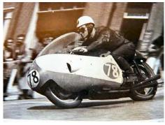
The race is underway and everyone is listening for the first sound of an engine, because this year we have multi cylinder engines. The Gilera 500cc 4 cylinder above was ridden by Bob McIntyre and he was the first person to break the 100 mph lap from a standing start, the sound of the engine had a terrific sound.
